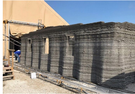
Fig. 2. US Armed Forces - 3D printed Barracks Image: Marine Corps Systems Command (MCSC)
